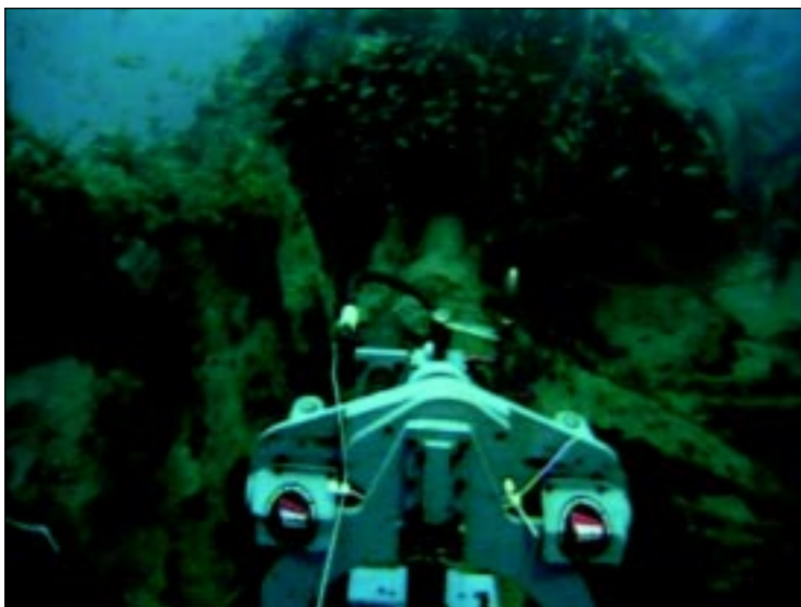
MONITOR's shaft looking forward with the Wach's guillotine saw in place around the shaft, ready for the divers to begin the cut.
