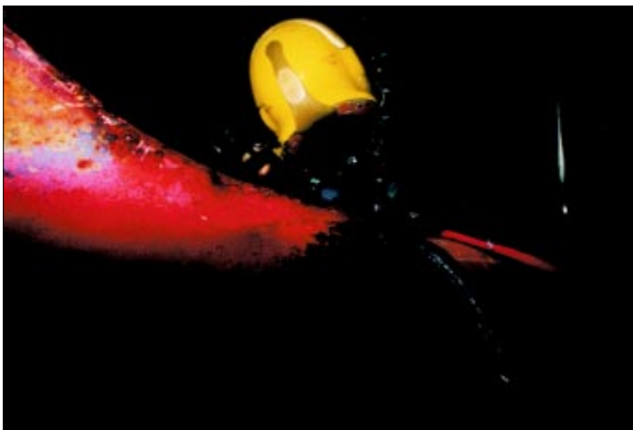
Welding rope guards on U.S.S. CALIFORNIA. Pictured RDL Site Bremerton Diver Dana Hershberger in MK-21 gear.
